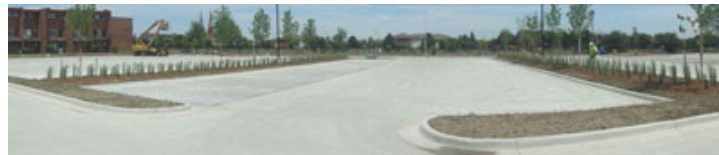
Pervious pavement within parking lots is helping leverage Detroit's 160-year-old utility systems by better managing stormwater prior to discharging it into the city's combined sewer system.
