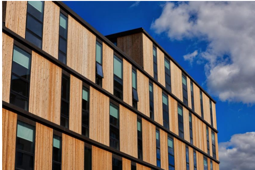
Each floor is wrapped with metal coping
