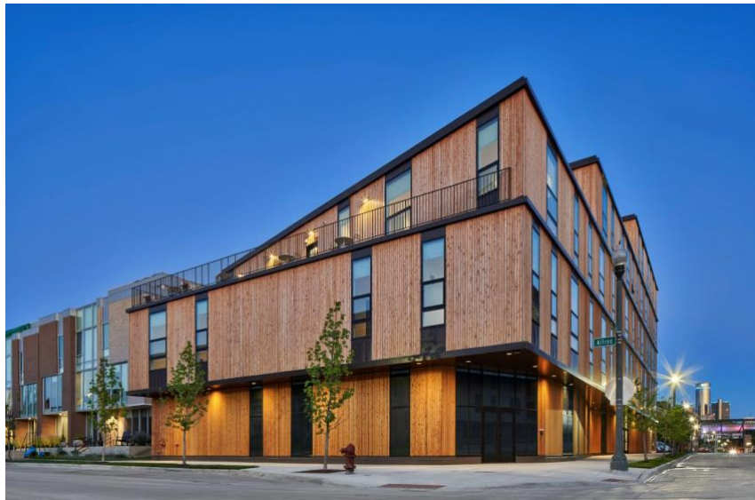
The apartment building by night
